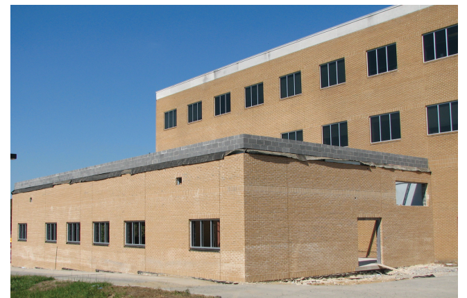
The $1.3 million wet labs addition to the TIC was funded by the Washington County Board of County Commissioners, Maryland Department of Business and Economic Development (DBED), and the Maryland Technology Development Corporation (TEDCO).
