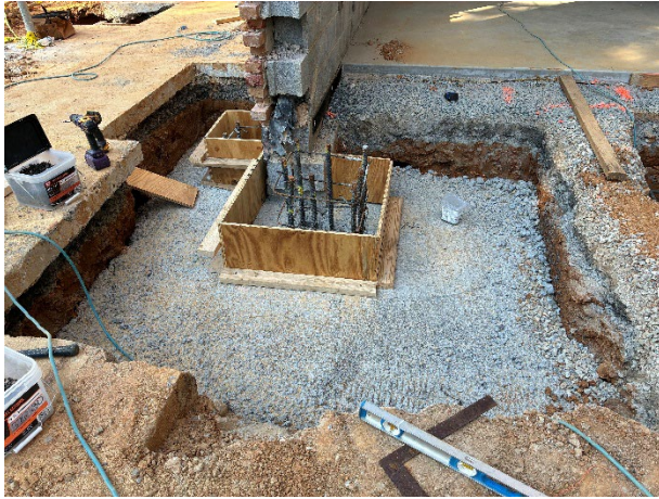
Footing and Foundation work
