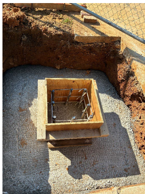
Footing and Foundation work
